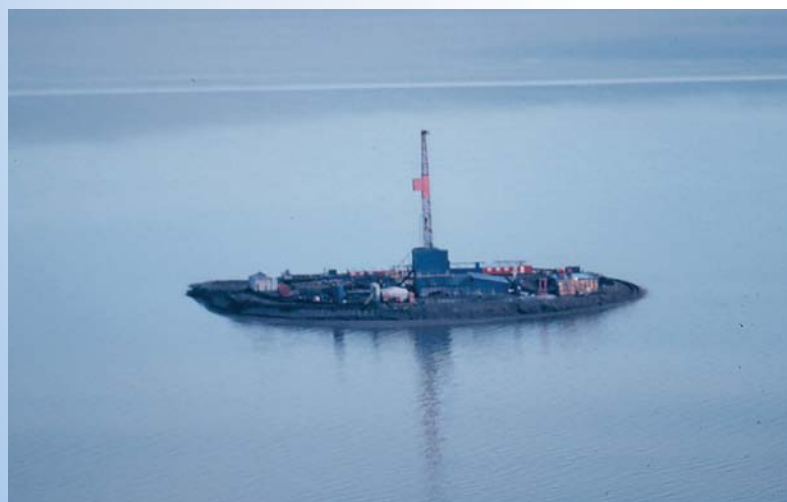
Offshore oil rig on artificial island, Alaska Photo: Captain Budd Christman, NOAA Corps/National Oceanic and Atmospheric Administration/Department of Commerce
